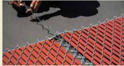
Insert the needle and connect the rolls same as regular chain link fence. Stand the fence up to the posts and top rail, loosely attach to the top rail, attach tension bar and stretch wire into place. **Do not cut the noodle until you have stretched the wire.**
