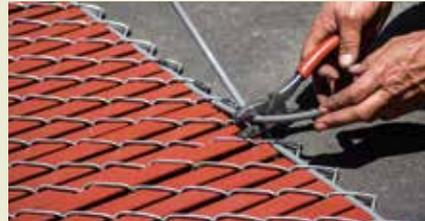
Cut the excess noodle halfway between the two selvages, so both ends touch and using the hog ring pliers hog ring both ends of the noodle to the wire.
